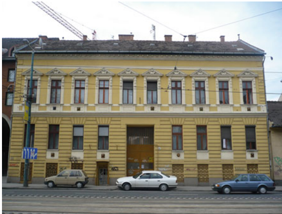
Fig. 3 Front view of the examined building
